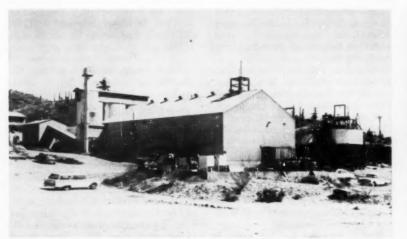
MINERAL HILL flotation mill, one mile from the shaft, is being revamped to handle over 1,000 tons a day of the harder Palo Verde copper ore.
